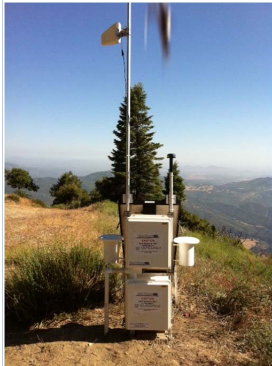
Palomar site installed in June, 2012
